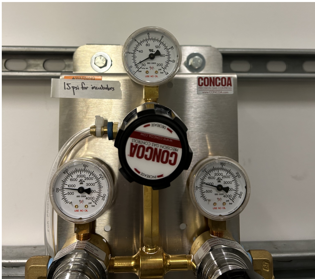
Fig. 5: Carbon dioxide knob (black, center) and pressure gauge (top, currently at 0 psi).
