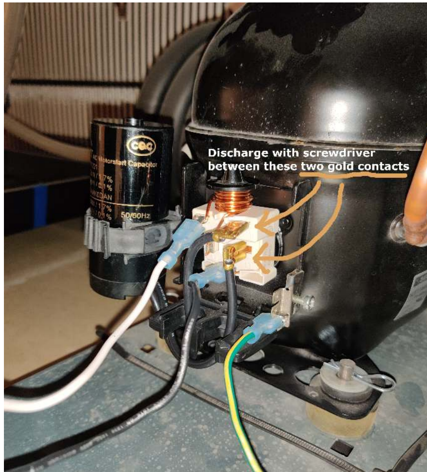
Fig. 13: Lightly touch a metal screwdriver between these contacts while only touching the plastic part of the screwdriver.
