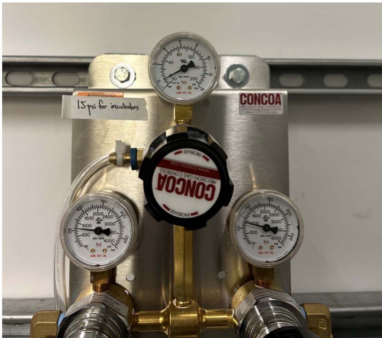
Fig. 6: Carbon dioxide knob (black, center) and pressure gauge (top, currently at 0 psi).
